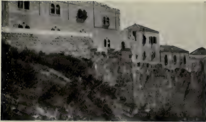
The Rampart Walk covered with 12 ft. of "tip," and showing a new wall built on top of the "tip."
